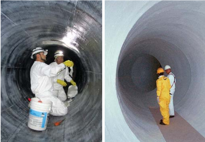
Installation and completion of the Tyfo® Fibrwrap® system
